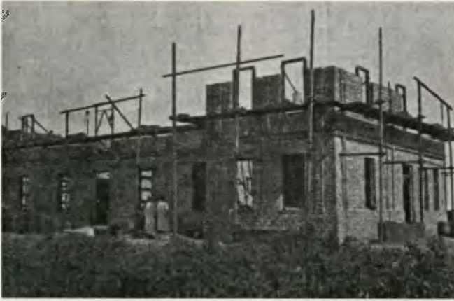
Construction of the sanitarium at Entre Rios continued only as quickly as funds were received to purchase the necessary materials.
