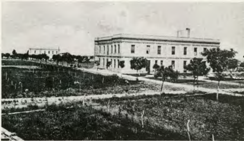
Both the college (background) and the sanitarium (foreground) can be seen in this photograph which was taken about 1917.
